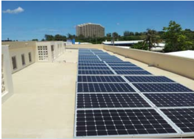
Photovoltaic (PV) panels are components of new construction projects. The GCC Annex facilities are intended to have a combination of rooftop PV for buildings and parking lot canopies. Walkways canopies outfitted with PV panels are also intended for the campus.
